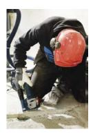
Figure 13B: Cutting concrete with HVLV extracted device (Source: Dustcontrol UK)
